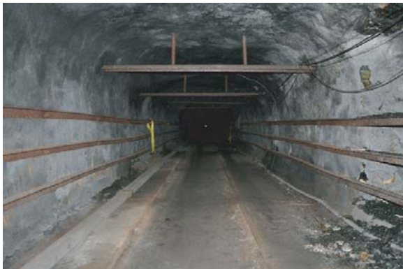
Figure 5. Bruceton experimental mine main entry.
