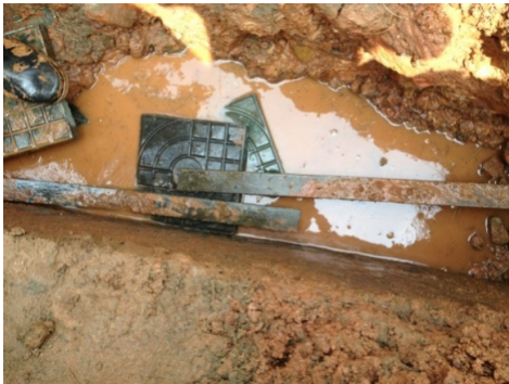
Figure 20. Disconnect branch.
