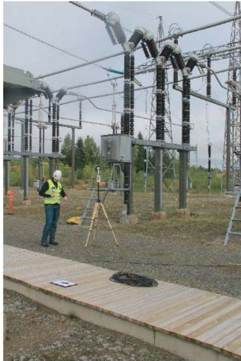
Figure 1. Preparing to measure the field strength using a Maschek meter on the passageway. On the right of the meter, there is a one-phase circuit breaker with three poles and six breaker heads. The breaker poles run approximately from northwest to southeast.
