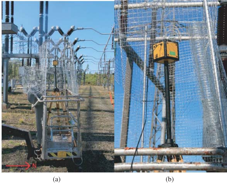
Figure 9. The position of the probe on the protected man hoist.
