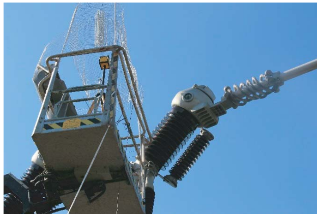
Figure 10. E -field measurements performed with the meter on the protected man hoist, with an opening in the net on a long side of the man hoist.
