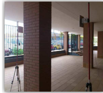
Figure 4. Picture of the studied column.
