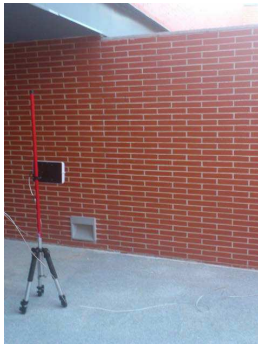
Figure 1. Picture of the studied wall.
