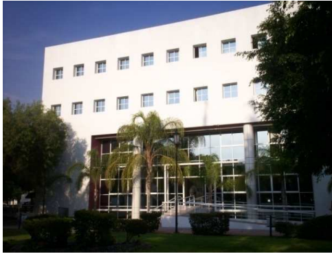
Figure 6. Engineering and Electronic Centre, Building 2.
