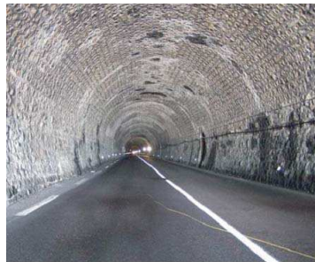
Figure 1. Straight road tunnel in which experiments were conducted.
