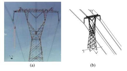
Figure 10. (a) Straight-line tower of  $400 \,\mathrm{kV}$  and (b) its numerical model.
