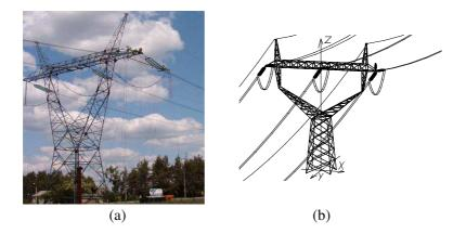
Figure 12. (a) Anchor tower of the 400 kV transmission line and (b) its numerical model.
