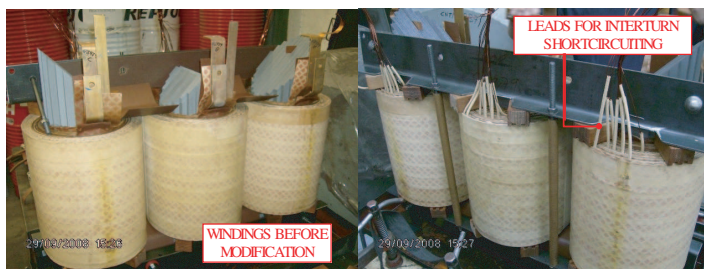
Figure 16. Modification of the windings for the installation of the short-circuit leads.
