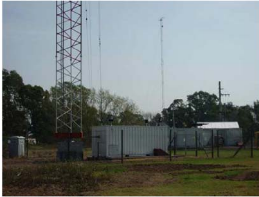
Figure B1. Picture of the monopole antenna of H = 197 m of height, and 790 kHz of frequency.
